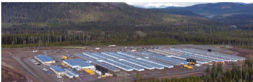
➤ Example of a temporary workforce accommodation that can house 700 workers.
